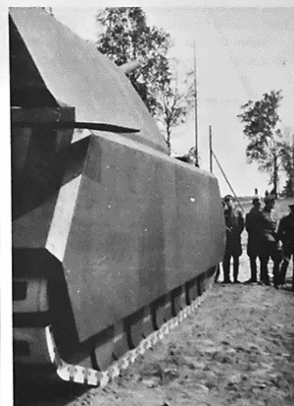
Above Right and Left: The full-scale wooden model of the Porsche-Maus on display for Hitler and entourage on 14 May 1943 still had a commander's cupola on the roof. In 6 decided that the Flammenwerfer (flame thrower) system (mounted on the right and left upper hull rear) would be dropped. (BSB)
